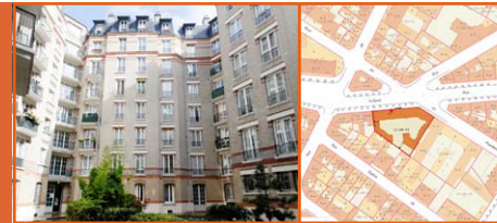
>>> (13 th ) >>> 207, Rue de Tolbiac >>> 1913-1922 >>> Public contracting authority >>> Architect >>> Georges Vaudoier
